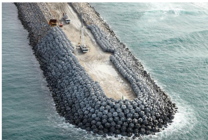
Outer harbour of Punta Langosteira (A Coruña, Spain), where Cubipod technology was used.
