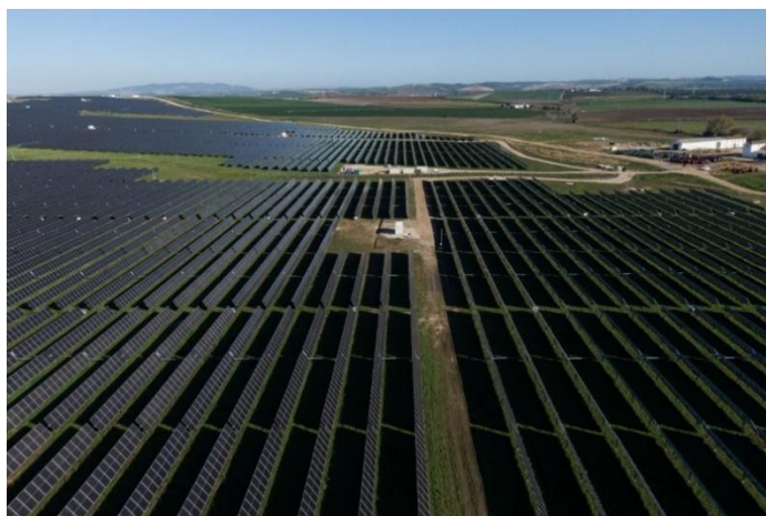
Photovoltaic plant developed by OHLA in Spain.
