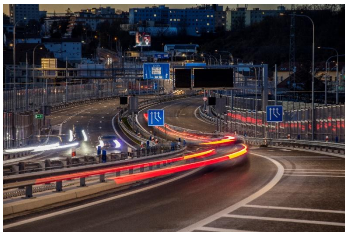
OHLA ŽS, the Group's Czech subsidiary, is one of the country's leading players in road infrastructure development. Pictured: the I/42 motorway, also delivered by OHLA.
