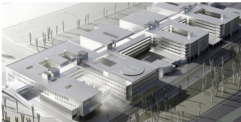
Development of the future Maternal and Child Hospital in Huelva, to be delivered by OHLA, with an estimated investment of EUR 82.6 million.
