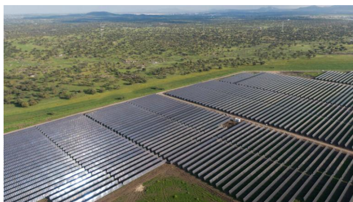
Photovoltaic power plant in Mérida, Badajoz (105 MW)
