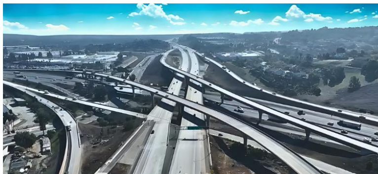
In California, OHLA USA reached a key milestone by opening all lanes to traffic in the SR-71 conversion to a freeway project, which was completed on schedule.
