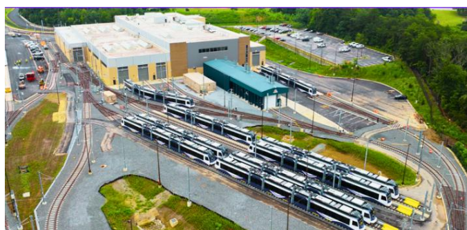
The arrival of the 28 light rail vehicles at the Purple Line's operations and maintenance facility, weeks ahead of schedule, marks a key milestone in the project's progress.
