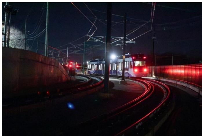
The Purple Line light rail, OHLA's largest project by value, during its testing phase.
