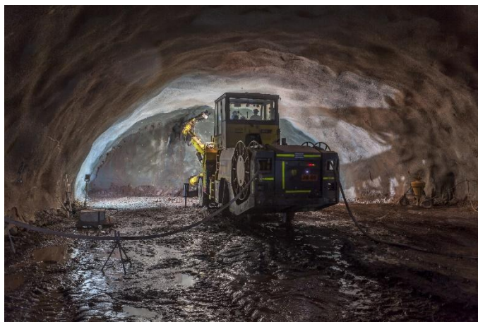
Machinery at work on one of the highways developed by OHLA in Chile.
