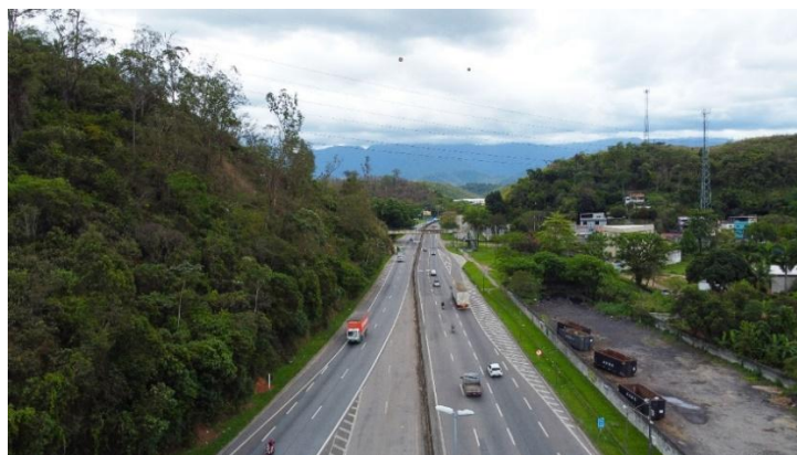
BR-040 federal highway, a concession brought into operation by OHLA in 2025, carrying more than 45,000 vehicles per day.
