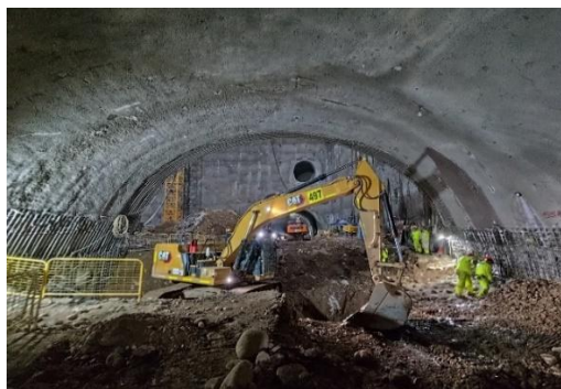
Machinery at work inside one of the tunnels on Line 7 of the Santiago Metro.
