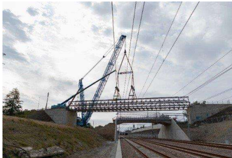
Removal of the 150-tonne Åkarp bridge in Sweden. Picture: Niclas Franzén, OHLA/NCC.
