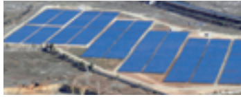
Mezzanotte Solar, photovoltaic plant in Lecce, Italy
