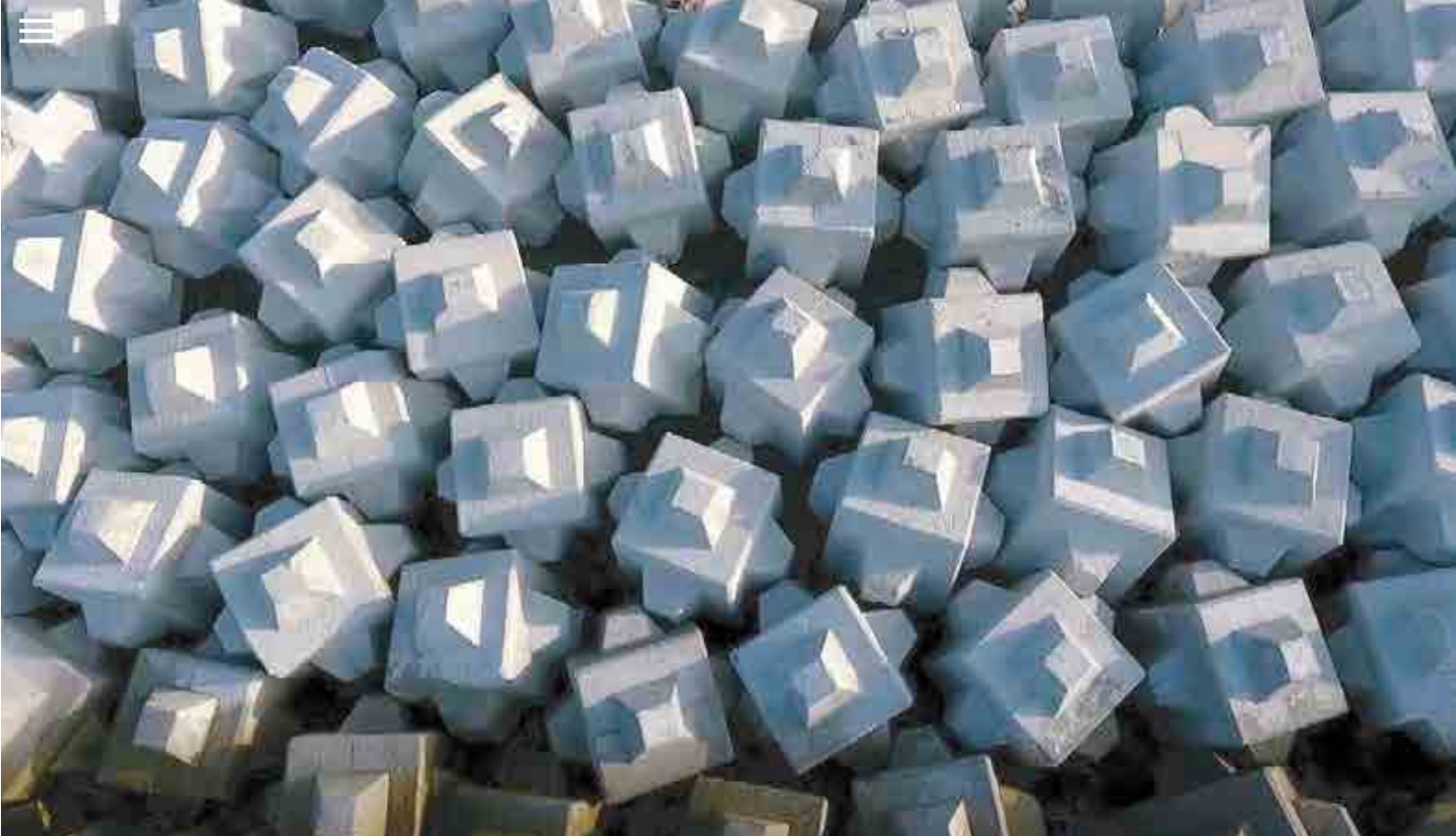
^ Acopio de Cubipods. España. Cubipods stockpile. Spain.
