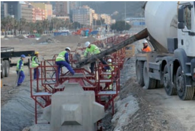
Hormigonado de cubípodos. Concrete filling of Cubipods formwork.
